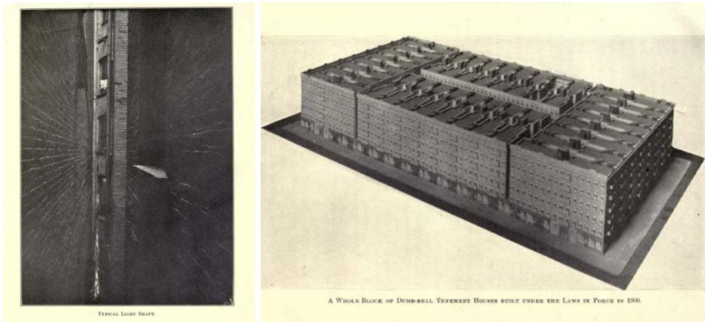
**Figure 10.** Narrow shafts resulting from the dumb-bell plan (DeForest & Veiller, 1903a; p.14&10)
